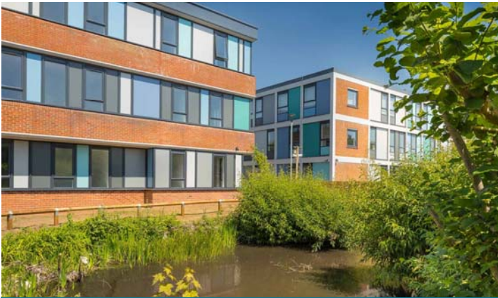
The former Nielsen offices in Risinghurst have been redeveloped as apartments, part of the Thornhill Park development Photo courtesy of the Shaviram Group
