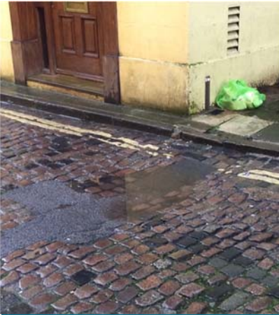
Merton Street – uneven cobbles, tarmac infill and yellow lines make for a visual mess and a danger to users
