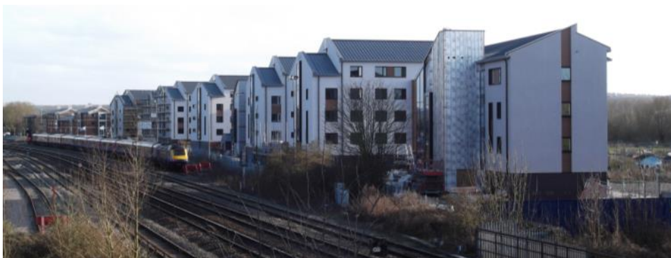
The scale of the Roger Dudman Way blocks can be seen from the railway lines. Their impact on Port Meadow, to the right, created a public outcry Photo courtesy of JP Bowen
