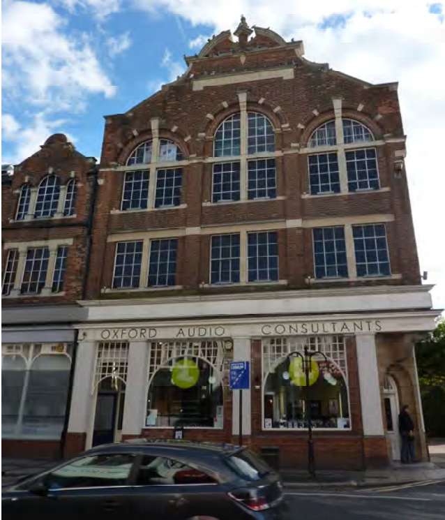
A recent OCS walk reminded us that many familiar buildings, like this one in Park End Street, owe their existence to the coming of the railways. This originally housed a furniture removals company.
